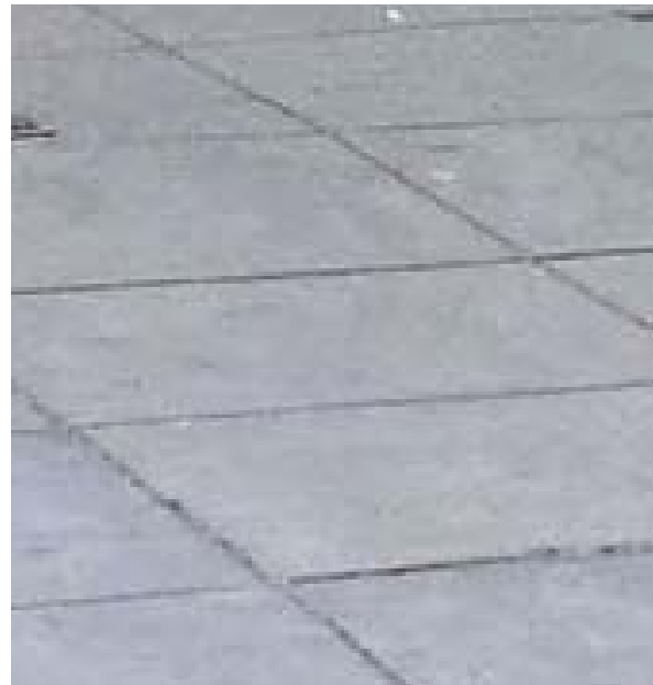
DC Standard Concrete Paving
